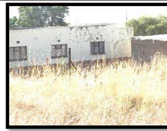
Photograph 3.12: Typical houses in the community, 29 May 2014
